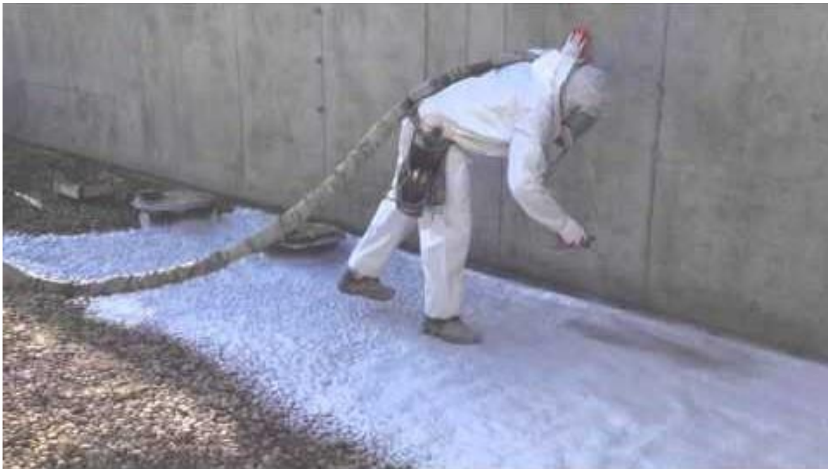
Slab Insulation Application
