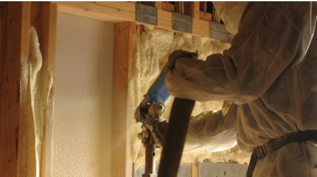
Interior Wall Application
