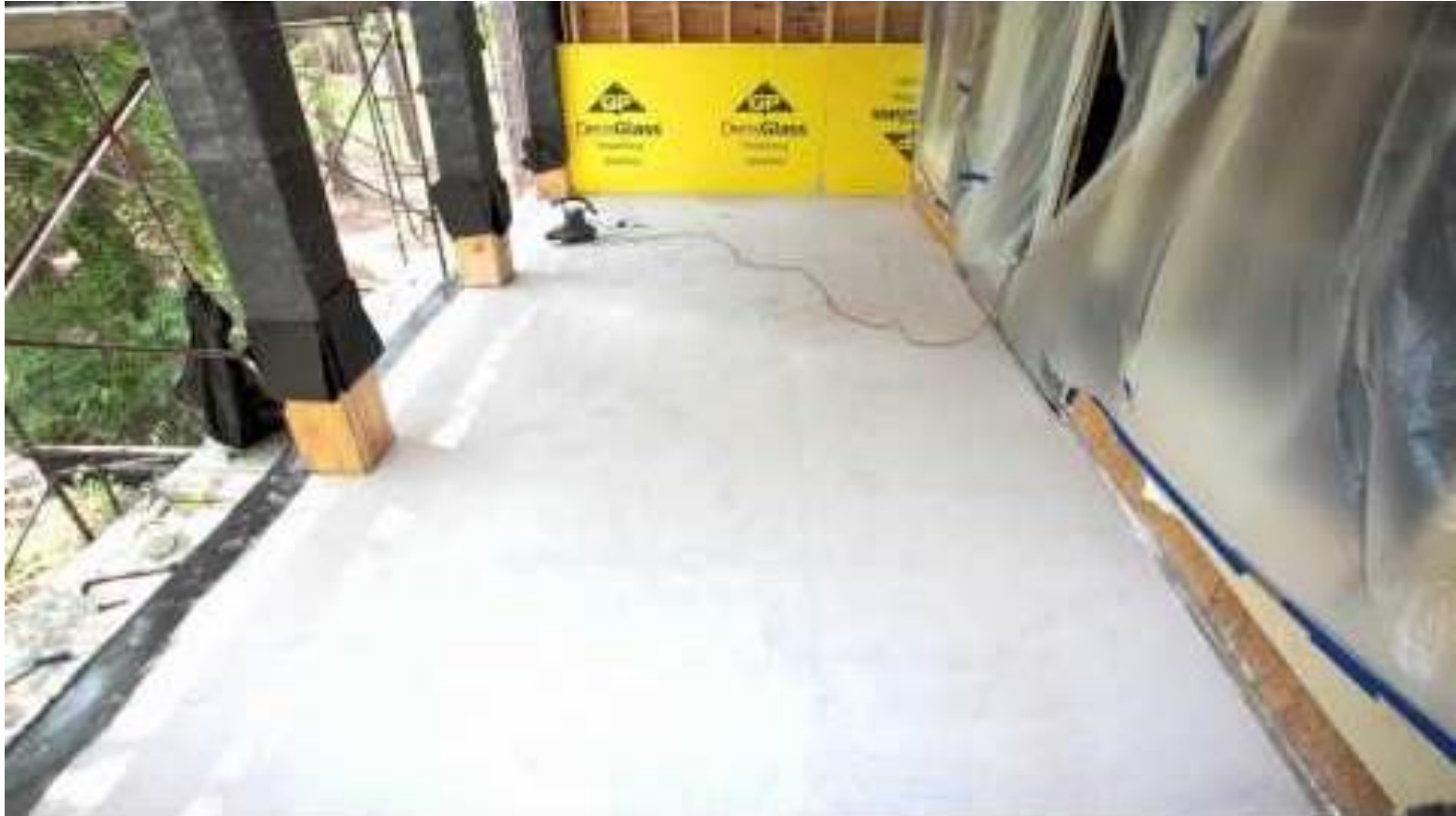
Polyurea Coating Application
