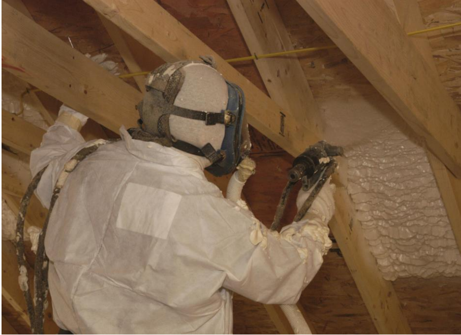
3" Average of Closed Cell Insulation
