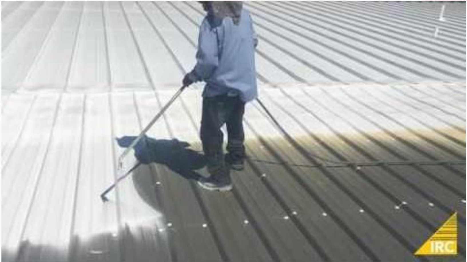
Metal Roof Restoration
