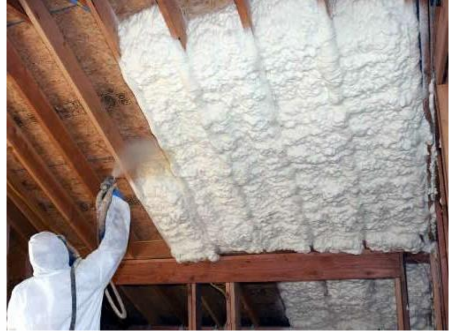
6" Average of Open Cell Insulation
